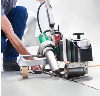
Welding modified bitumen
