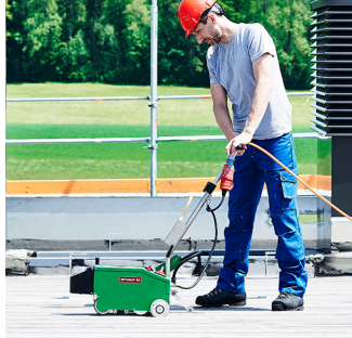
Overlap seam welding
